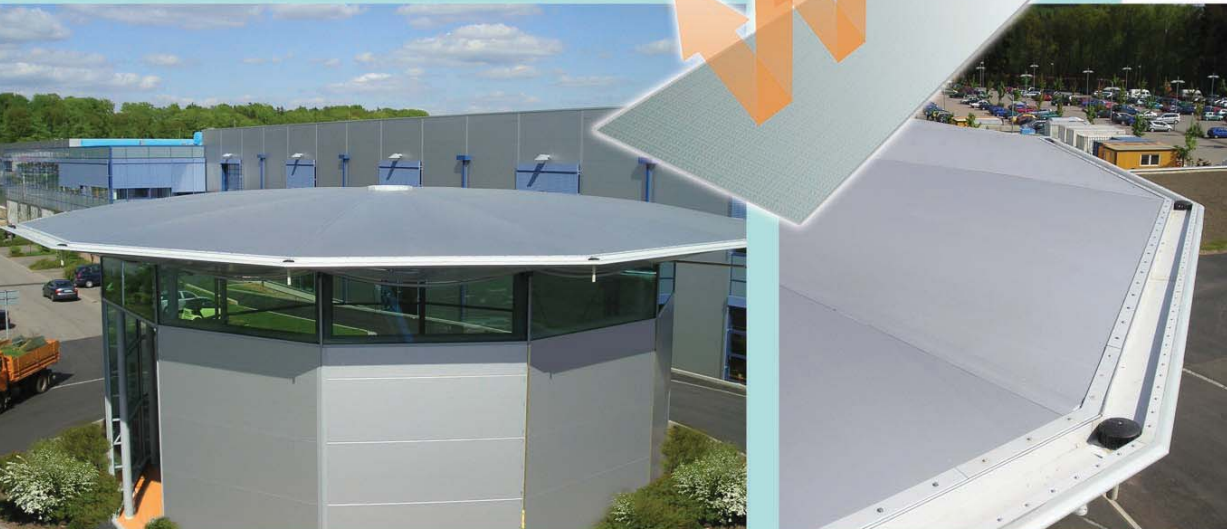
Fuel cell building, Festo-Rohrbach
